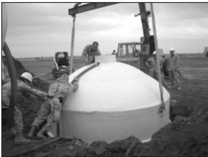
Installing water supply tank for the Firedawgs
